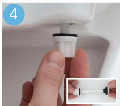
4. Mount the cistern firmly / Montera fast cisternen
